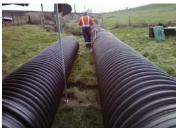
Pipe relining for culvert reinstatement
