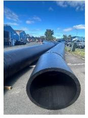
Left – Some large SOLID WALL pipes prepared for installation in a WWTP, and
