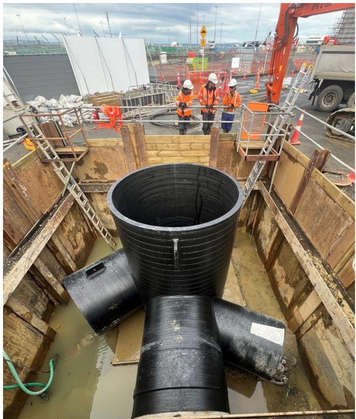
Fig 2. Airport manhole known as the 'turret'
